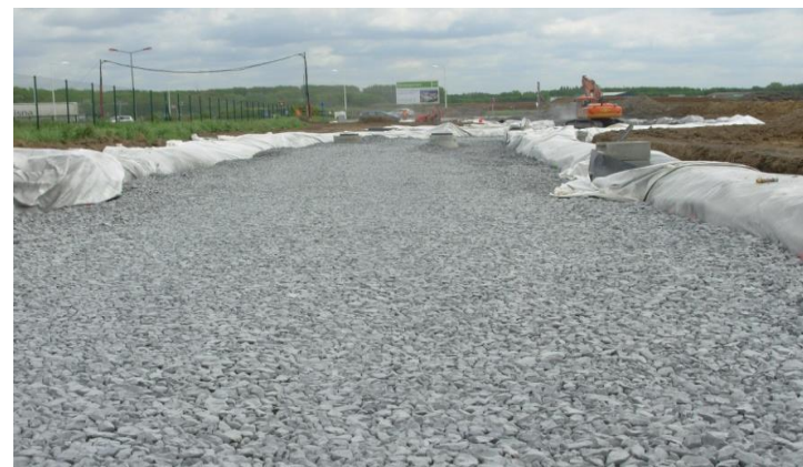
Infiltration reservoir roadway with classical asphalt
