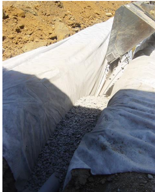
Filled with stone (Void ratio: 35%)
