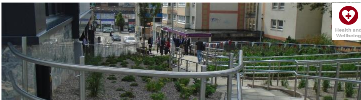
Figure 16: Plymouth City Council's First SuDS Pilot Site at Market Way and Mayflower Street
